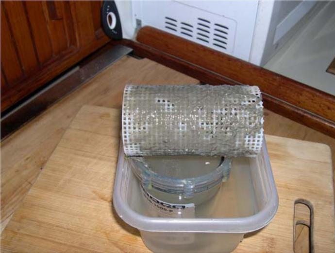
There's always maintenance work, such as cleaning out filters. This one is on the water feed to the heat exchanger for the air conditioner. Ugh !
